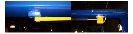
**4.** Run electrical cord into the beam and back out of the column using provided bulk head fittings.
